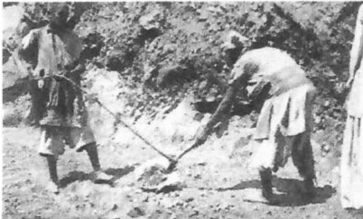
TWO-MAN SHOVEL.—Road-mending made easy: one man digs the shovel in, and the other helps him to lift it and its contents by means of a rope tied to the handle.
