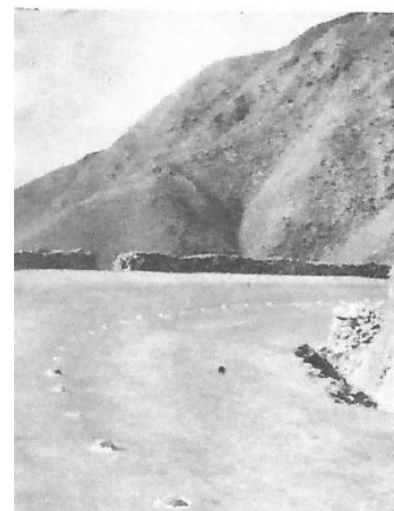
INDICATORS. — Raised white stones make a psychologically good central road division, and their use on blind corners of the Malakand Pass has proved more effective than white lines. The idea is also used in parts of the English Lake District
